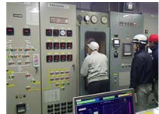
On-site inspection at Kumamoto Plant, Japan
