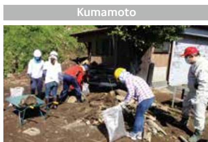
Volunteers removing dirt and wreckage in a residential area
